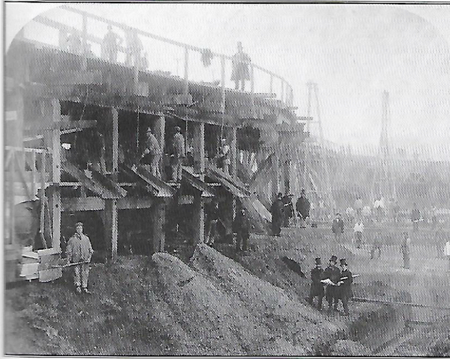
The concrete mill at Crossness, 1865. The Southern outfall sewer may be glimpsed in the distance. (Thames Water plc)
